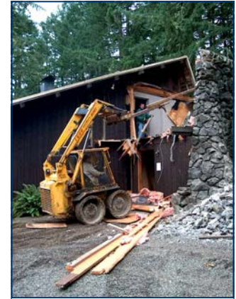
Dec. 04 - Demolition of old Lodge entry.
