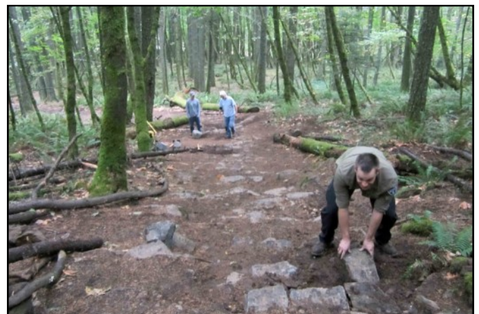
Putting in rock steps during September trail maintenance—Photo by Pat Soussan
