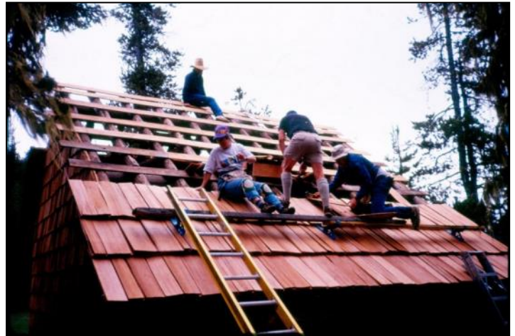
Last day: installing shakes on the back roof.
