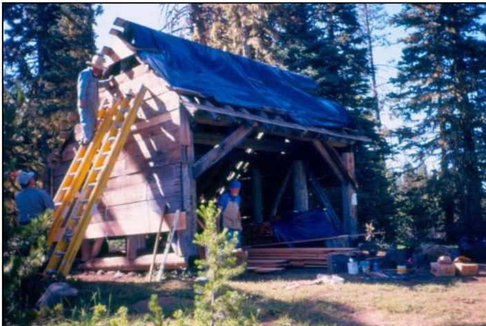
First day: hanging new shiplap on the north wall.
