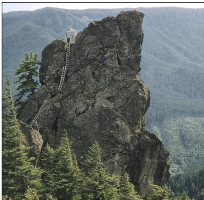
Rooster Rock photo taken by Obsidian Bob Medill in 1961 shows the deteriorating ladders that once provided access to the pinnacle fire lookout on top.
