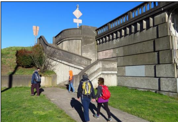
Access to the bridge at the north end.
