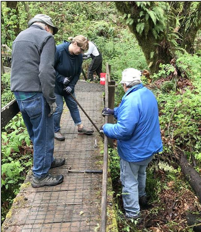
Clara, Dave and Jennifer start demolishing the railings.
