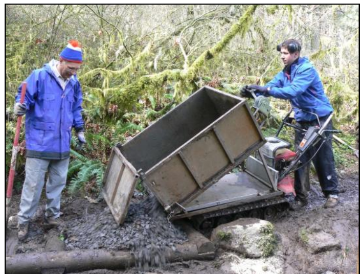
Jim & Peter building trail at Spencer Butte
