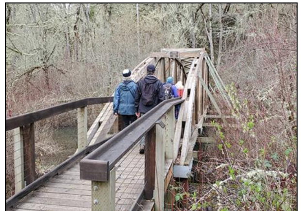
4. Crossing Adkison bridge.
