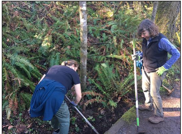
Jennifer and Lynn digging out a culvert.
