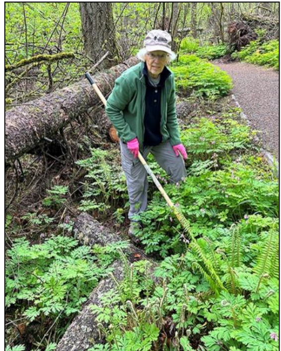
Janet amongst bleeding heart plants that are blocking a culvert.
