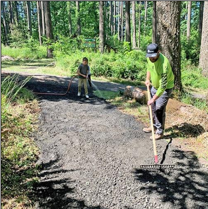
Matt doing a final raking with his son Naith watering the gravel before compacting begins.
