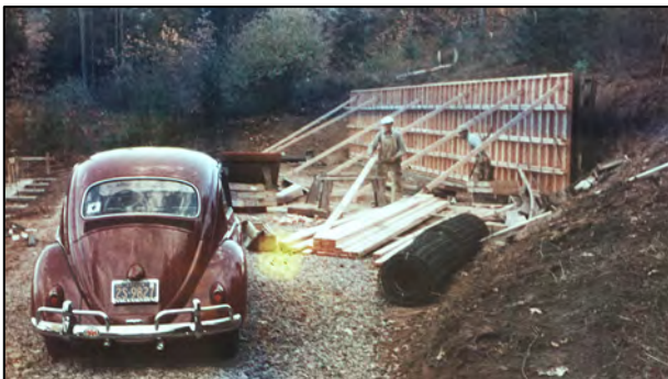
The back wall goes up October, 1960.
