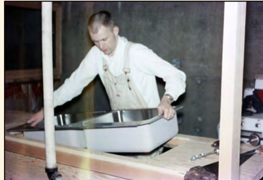
Tom installing the sink in the Lodge kitchen.
