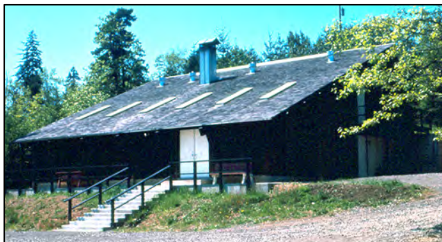
The concrete porch and stairs were completed on the east side of the Lodge in May, 1964. The look of the east side has remained relatively unchanged since then.
