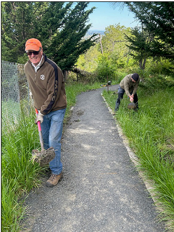
David filling a scour in the tread while Matt clears a drainage ditch.
