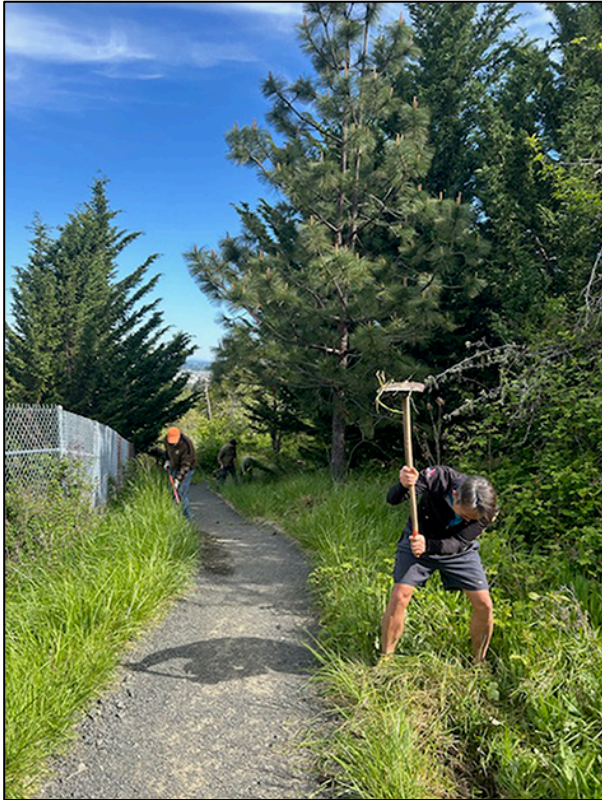
Sony swinging hard to reestablish the drainage ditch through heavy grasses.
