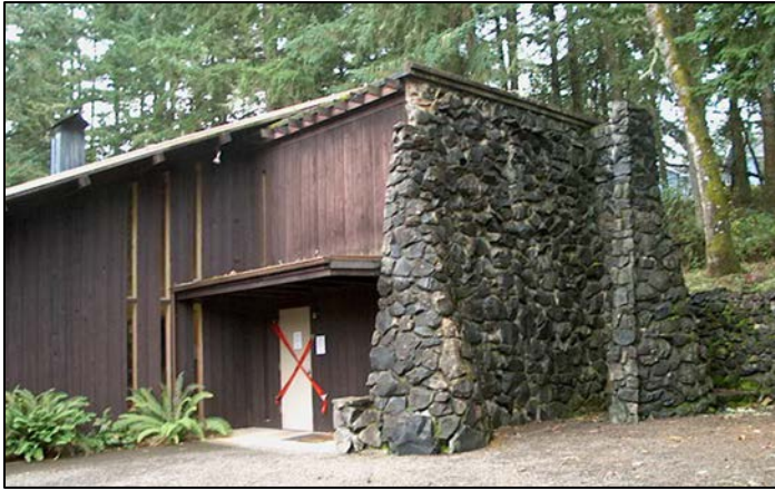
Lodge with danger warning on entry door. Photo by John Jacobsen.
