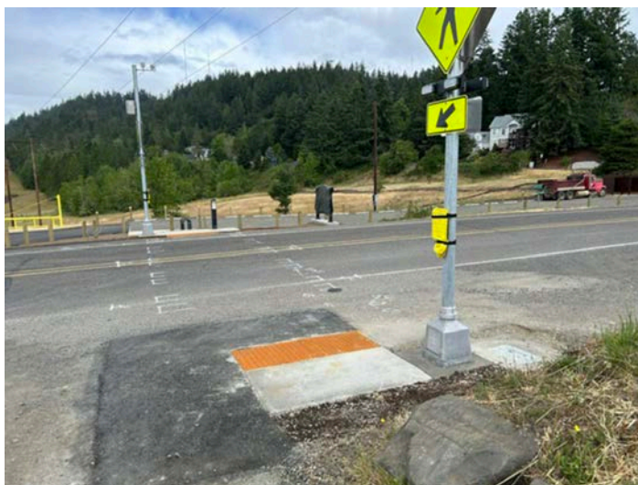
Safer crossing of Willamette Street, between the old Willamette & 52 nd lot on the east side, and the new SEM parking lot on the west, is in the works.
