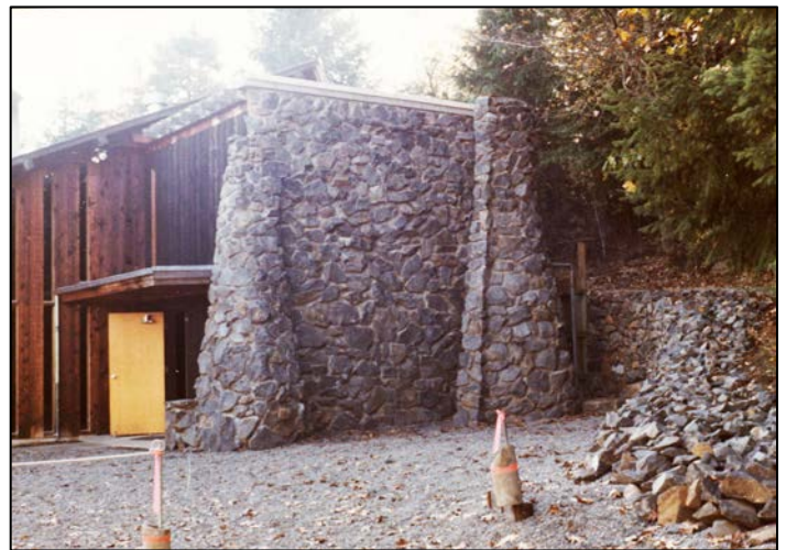
Completed Wall. Photo by Mary Castelloe.
